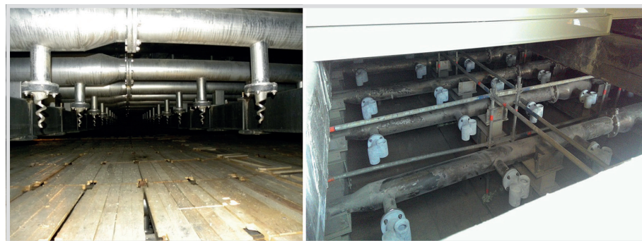
Fig. 4. Replacement of old helical nozzles with tangential bi-directional nozzles (reusing the existing spray lances, turned thru 90^\circ ).
