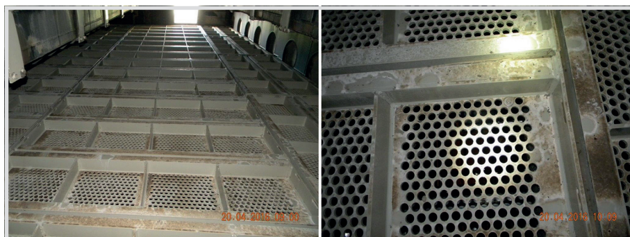
Fig. 7. Tray level after about 8 months of continuous operation.
